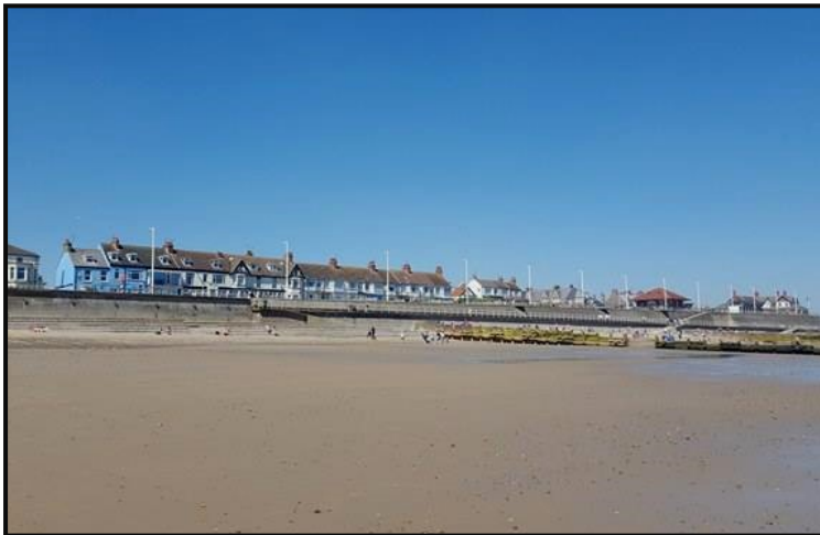
Figure 1: A view from the sea end of a groyne back to the sea wall and splash wall.
